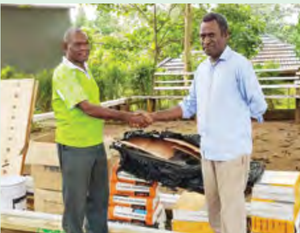
Vanuatu Central Hospital – Children's ward upgrade.
