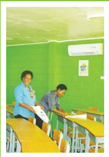
RENOVATING LIBRARIES & CLASSROOMS
