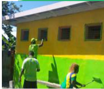
RANADI Lunga School Ablution Block renovation
