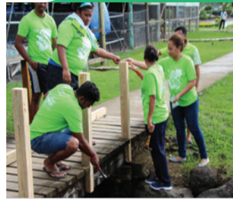
SAVUSAVU BRANCH Maintenance and refurbishment of bridge walkway
